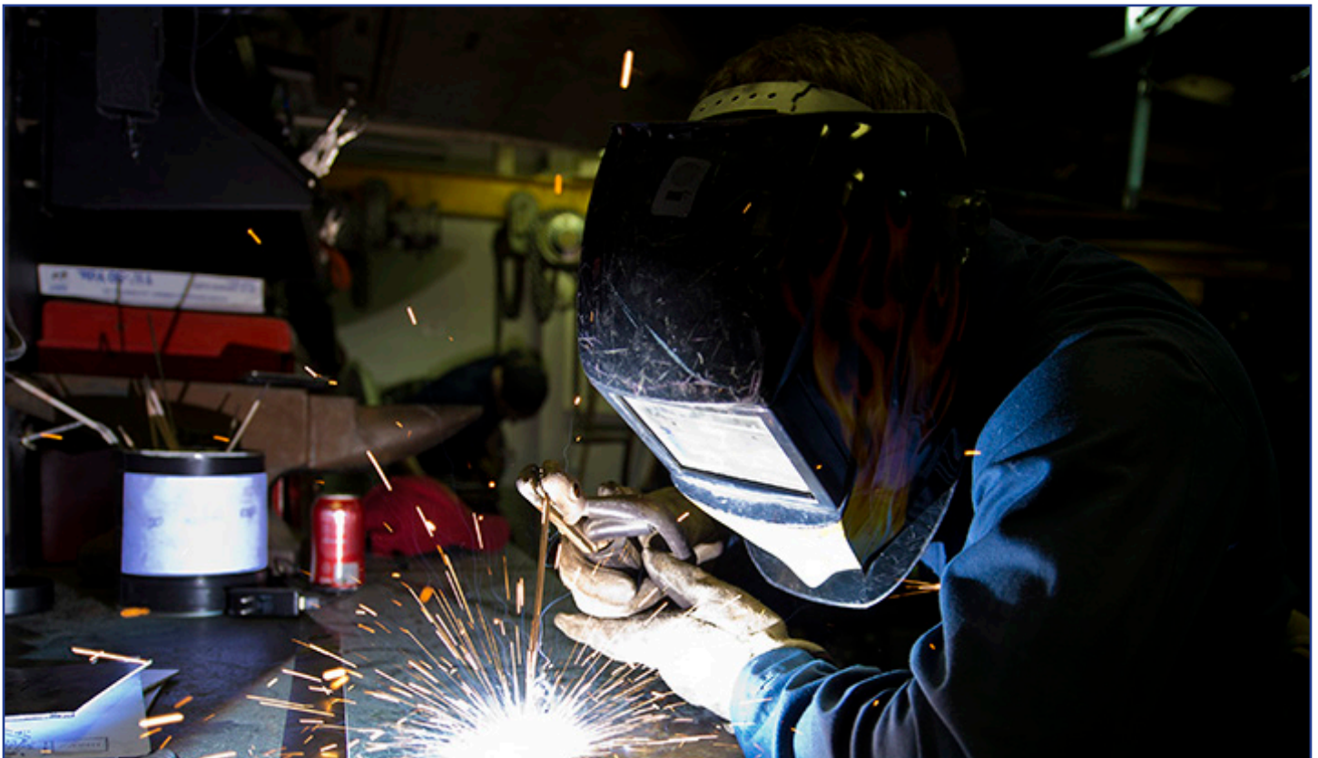
Hull Maintenance Technician 3rd Class Jesse Belfi strikes a welding rod to mend the hinge of a quick-acting watertight door handle aboard the USS Bonhomme Richard (LHD 6). U.S. Navy image.
